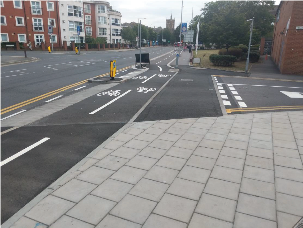
Figure 11 - New continuous footway/cycleway at junction in Kingston - Source: Kingston Cycling Campaign
